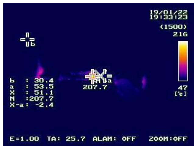
Figure 4.3: Heat generated from 4.00A Arc-fault.
