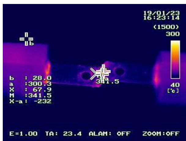
Figure 4.6: Heat generated from 8.33A Arc-fault.
