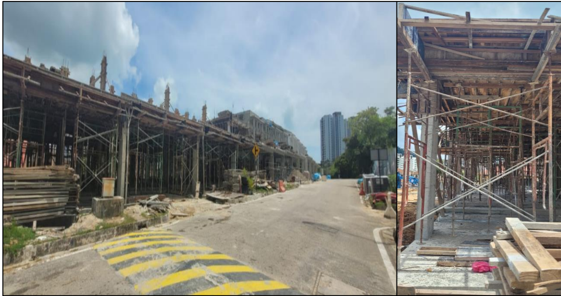
Figure 4.11: Project site with no safety hoarding or fencing (Corp. J)
