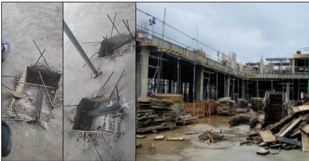
Figure 4.14: Project site with no safety label or barrier for the exposure reinforcement bar and poor site cleanliness (Corp. H)
