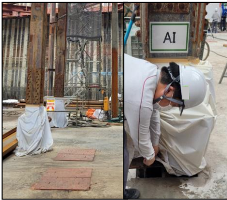
Figure 5.11: Plastic sheet to prevent fire
