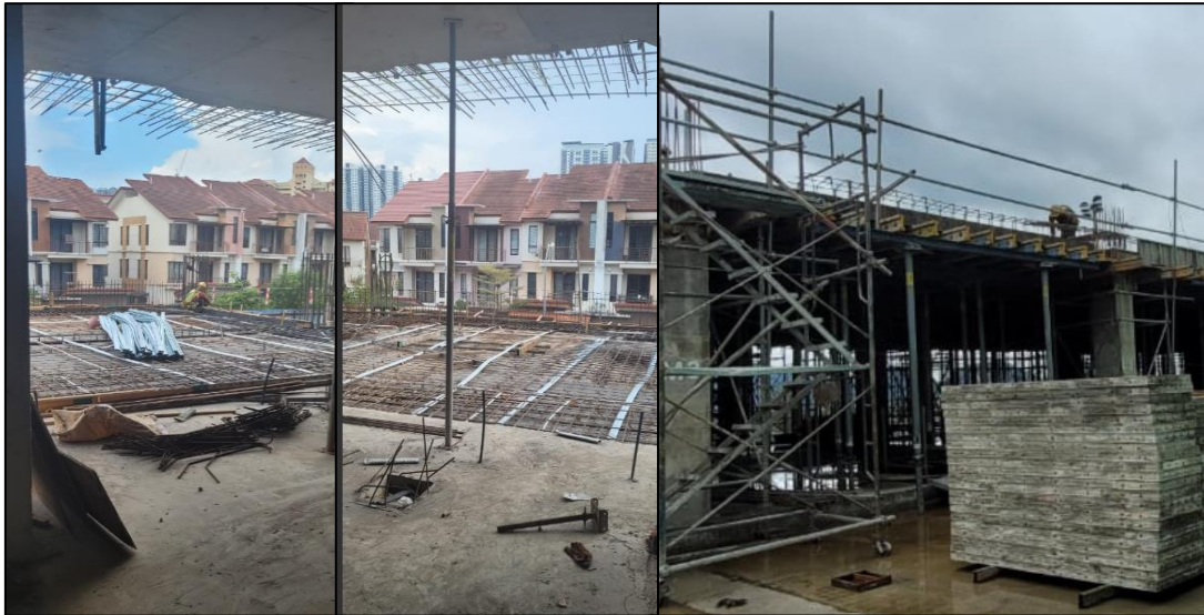
Figure 4.13: Project site with no safety netting, scaffolding is not proper installed and worker is not wearing PPE (fall prevention) (Corp. H)
